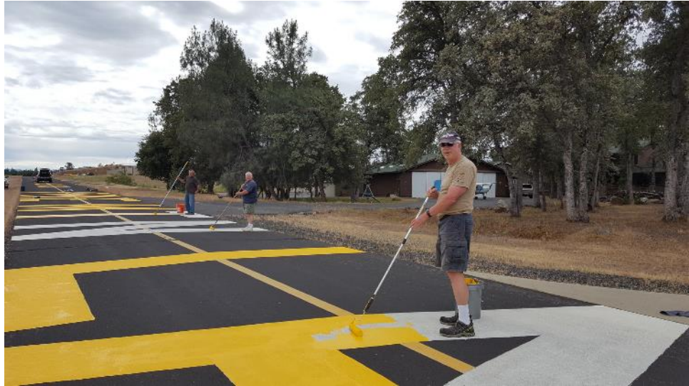
Volunteer Project - Painting the taxiway markings yellow
